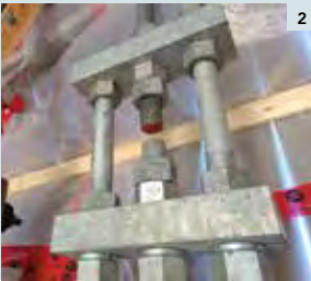
2. Splice detail of the vertical steel tension rods. See drawing far right.
