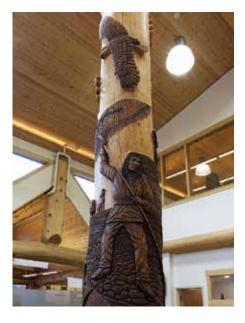
building was engineered in massive (solid) wood components. The log posts and beams, up to 40 inches in diameter, carry all the loads, from the SIP walls and roof panels through to the foundation. Emphasis was placed on structural wood joinery and minimizing the metal fasteners required.
