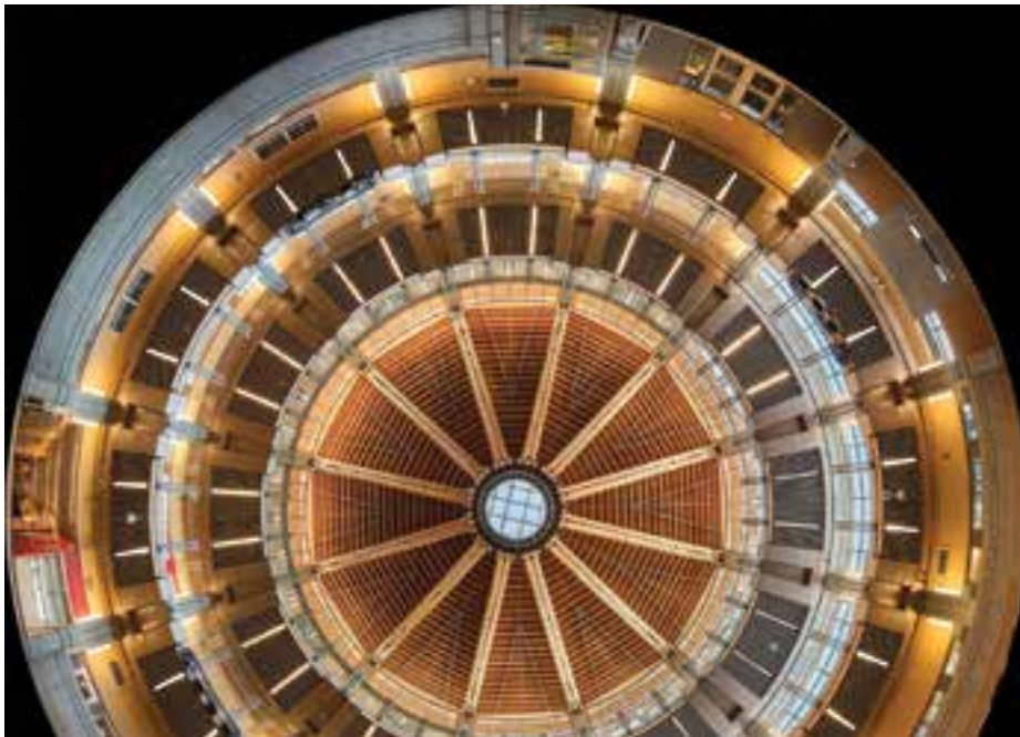
ABBOTSFORD SENIOR SECONDARY SCHOOL PHOTO CREDIT: AARON MILLAR, CRAVEN | HUSTON | POWERS ARCHITECTS
