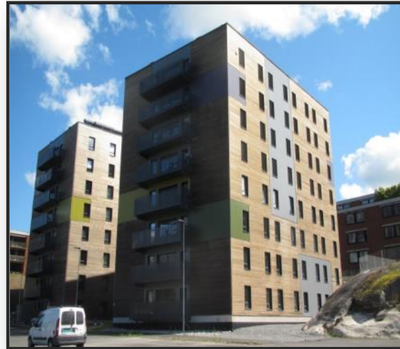
2 @ 8 storeys CLT buildings, Oslo, Norway
