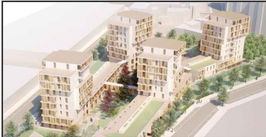
4 CLT residential buildings/social housing @ 9 storeys, Milan, Italy
