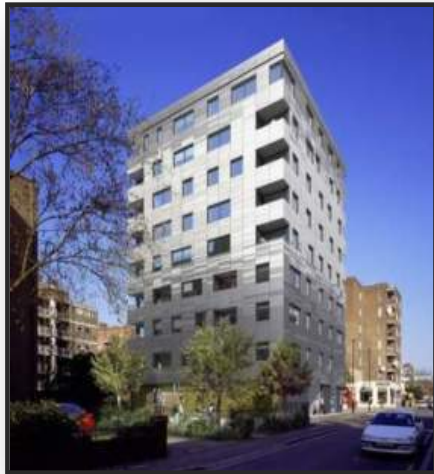
9-Storey buildings, London, UK 1 st storey concrete, 8 storeys CLT
