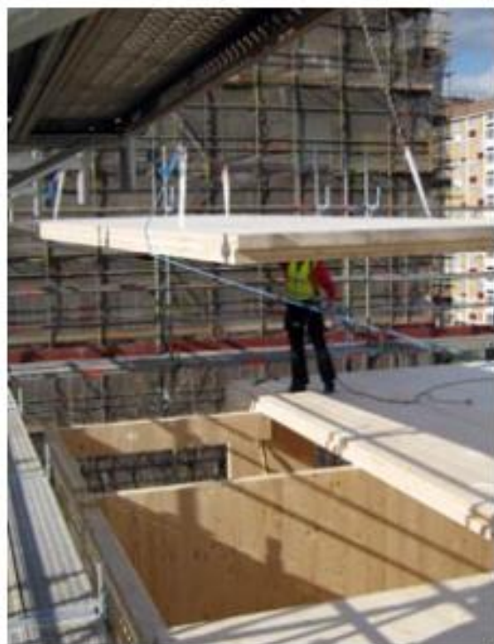
Floor panel installation.
