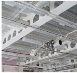
2. Steel Truss Girders
