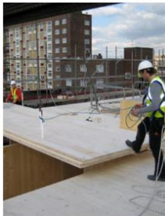
Floor panel installation.
