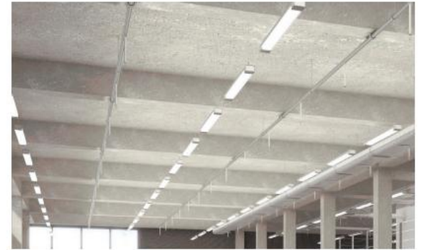
4. Reinforced Concrete Beams & One-Way Slabs
