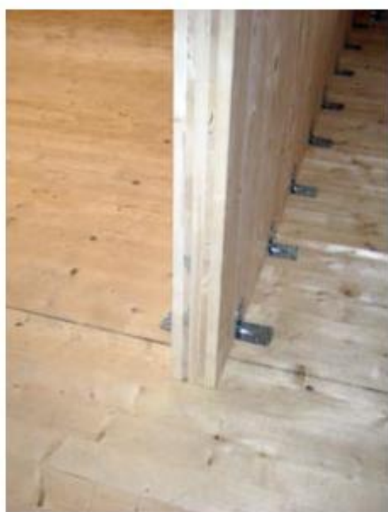
Wall panel anchored to floor panel.
