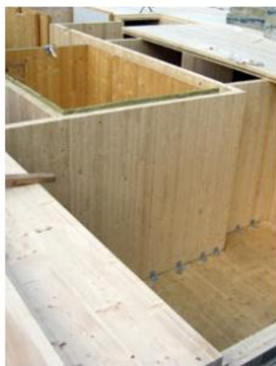
Typical internal wall arrangement.
