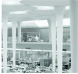
1. Reinf. Conc. Cant. Slab
