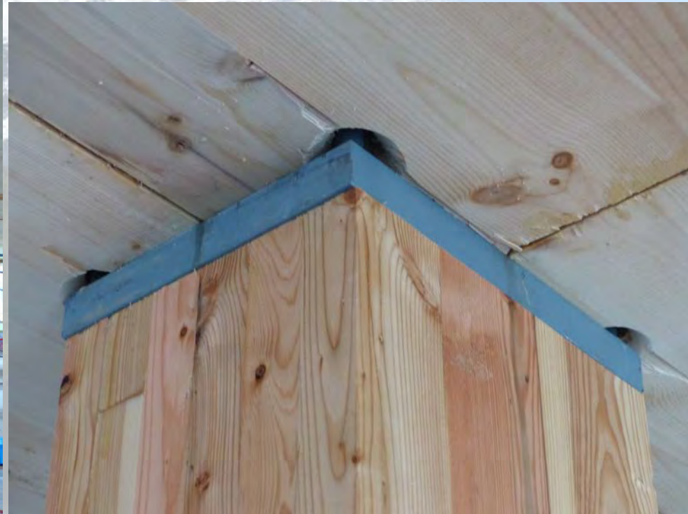
Connection at junction of 4 CLT panels
