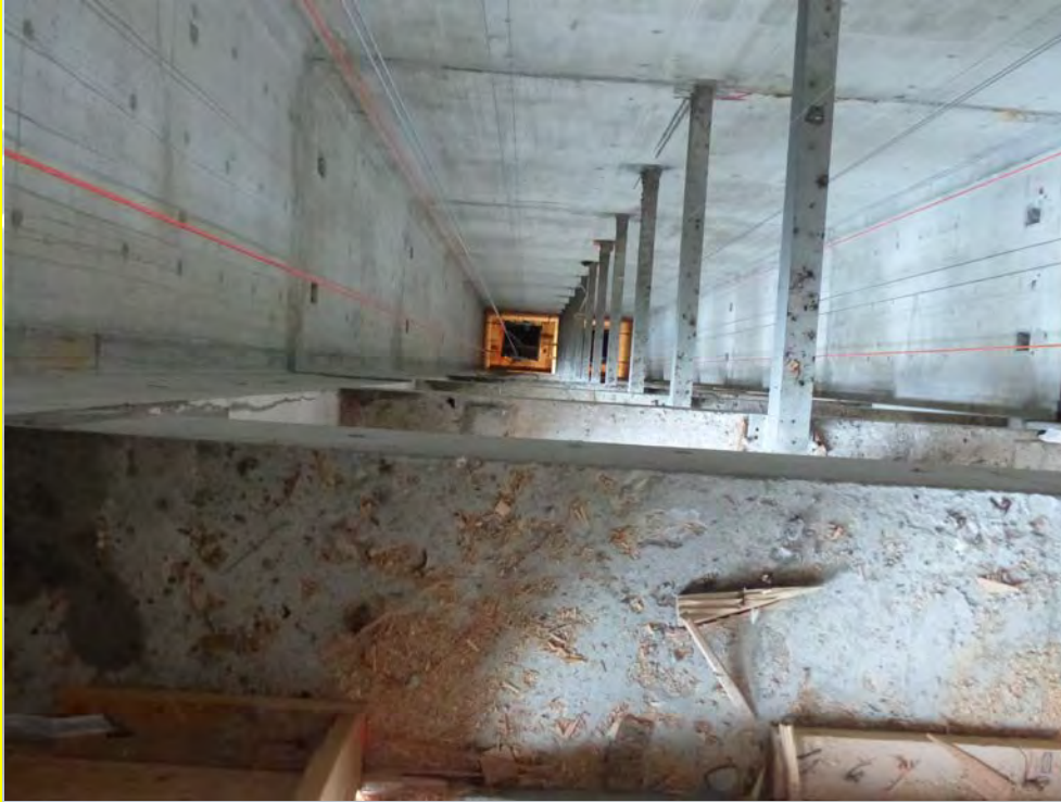
Concrete Core elevator shaft
