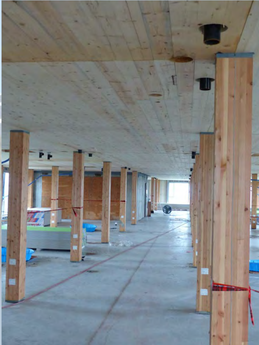
Exposed wood before Drywall
