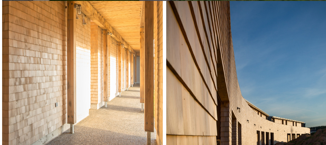
Cabot Links Lodge (Nail Laminated Timber) Architect: Fowler Bauld & Mitchell Ltd. Photo Credits: Greg Richardson Photography
