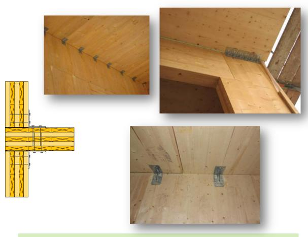
Most commonly used connection system in CLT assemblies in Europe & Canada
