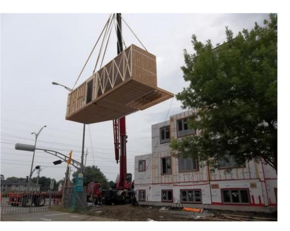
Modular construction may not be as economical as we thought, because of the extra structure required for the ceiling of the units during transport and installation, and the difficulty of access for all the interconnections required for structural integrity.
