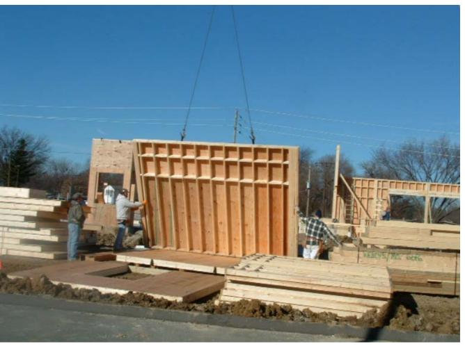
But you definitely need to use prefabrication of walls and floor sections.
