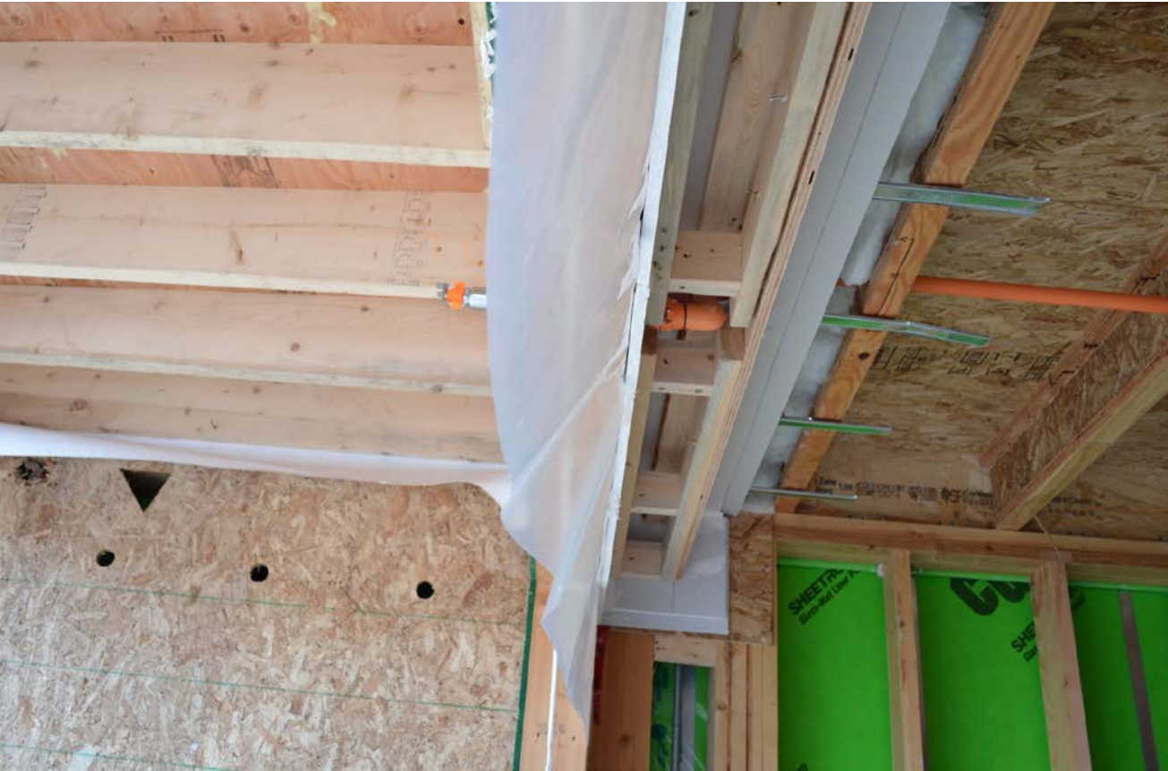
Sprinklered protection at underside of balconies
