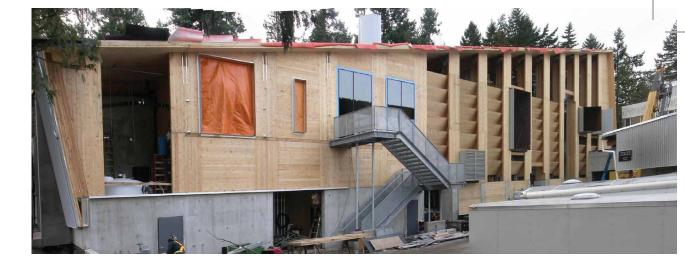
design, and showed air intake on the low windward side, and air exhaust on the high leeward side. As well, horizontal, outwardly angled CLT panels helped direct heat upwards and away from the power plant towards the glazed areas where heat could be conducted to the exterior. These panels also encouraged a convective flow to mitigate the formation of condensation on the glazing.
