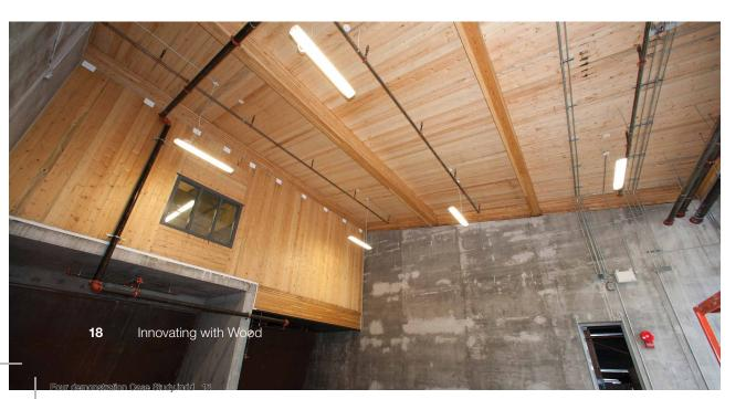
The introduction of CLT panels to North America provides architects and engineers with more design options and a more sustainable building system for heavy structures; one that displaced applications normally relegated to concrete or masonry. This highly promising wood system has been identified by the forest products industry, as well as the research and design communities, as a new and innovative opportunity for advancing wood in non-traditional applications.
