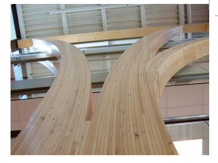
A third party consulting company with expertise in building code and fire protection was hired to develop a proposal for an alternative solution to demonstrate, through the use of empirical data, that heavy timber (glulam) could be used throughout the atrium. In the end the atrium consisted of heavy timber and acted as a separation between the existing building and the new development at the third-storey. The glulam was supplied by Western Arch Rib (Manitoba).
