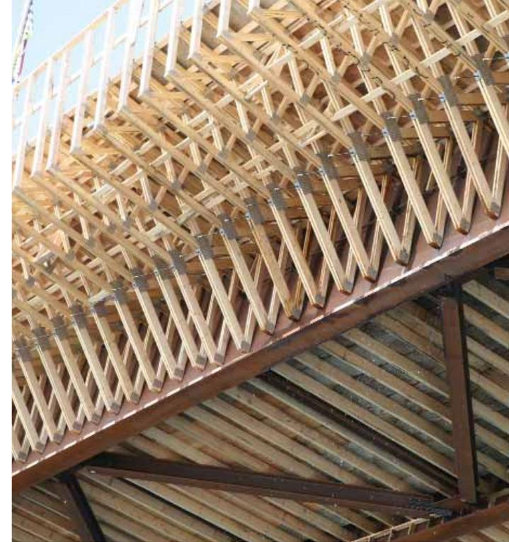
Reclaiming the usable lengths and gang nail plates was investigated as an option for the trusses on completion of the project, but was found to be uneconomical given current market conditions for wood products and available labour in the area. Instead, the trusses will be economically disposed of and the wood fibre recycled.▲
