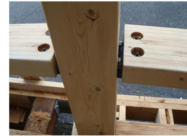
The structure is designed with simple connections to be completely demountable, enabling the material to be recovered for future use with no loss of structural value.
