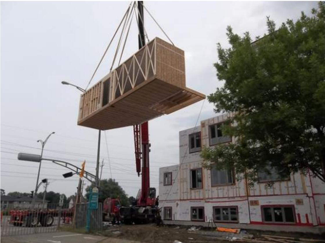
Modular construction may not be as economical as we thought, because of the extra structure required for the ceiling of the units during transport and installation, and the difficulty of access for all the interconnections required for structural integrity.
