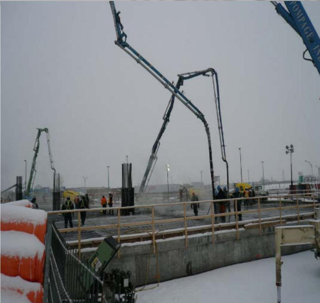
Then the concrete freezes if we don't heat it with a temporary tent. So we have to fight with the contractor to get him to heat and cure it properly, and we keep the temporary wood structure in place, and it gets in everybody's way for a month or two so we can slow the pace and make them suffer.
